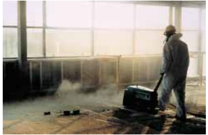
This industrial process (scabbling) generates a lot of dust. Formal measurements showed that respirable dust and silica levels were several times in excess of those advocated in British standards. The highest exposure arose during sweeping up
