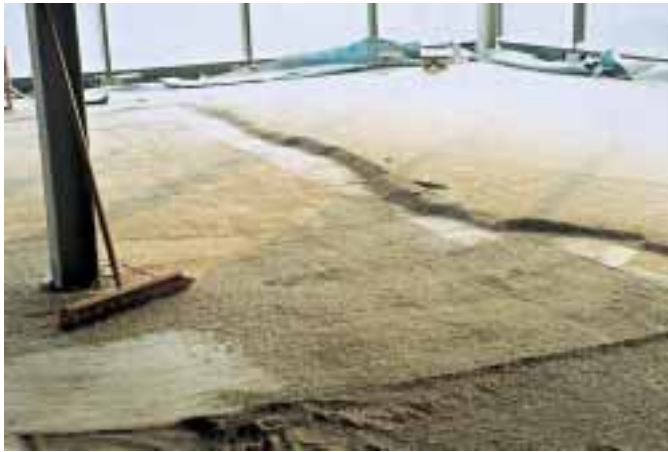
This industrial process (scabbling) generates a lot of dust. Formal measurements showed that respirable dust and silica levels were several times in excess of those advocated in British standards. The highest exposure arose during sweeping up
